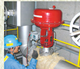
Overhaul of diaphragm valves
