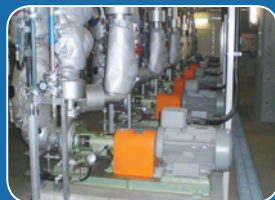
Maintenance of Pumps, Blowers, and Compressors
