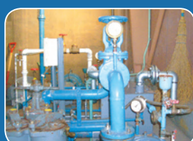
Installation and maintenance of water supply and sewerage equipment
