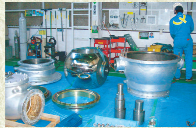
Overhaul of ball valves
