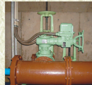
Inspection and adjustment of motor-operated valves
