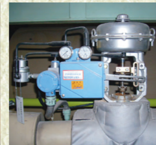
Overhaul of control valves
