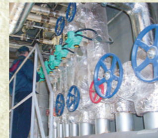
Installation of butterfly valves
