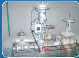
Maintenance of Various Regulating Valves
