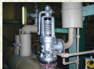
Installation of safety valves
